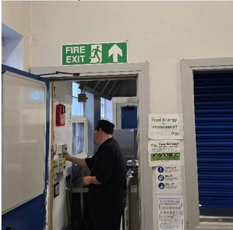
The fire exit signage at the far end of the corridor is duplicated following the addition of new bulkhead emergency lights. It would be more presentable if the old signage was removed – as this may pull the paint off, wait until the area is next due to be painted.
