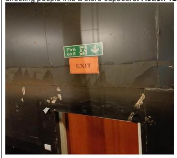
The emergency exit sign placed on the emergency light fitting above the exit door in the main hall should be removed as this door in no longer in use as an emergency exit. **Action 12.2**
